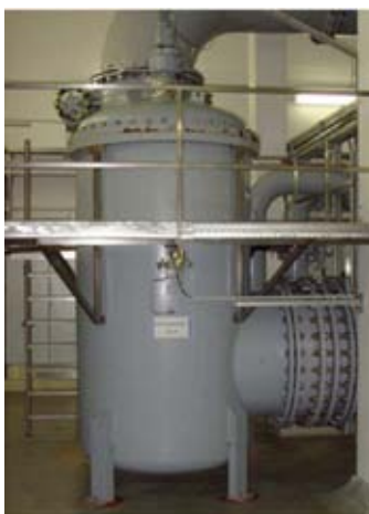
BOLLFILTER Automatic Type 6.18 System at WAG Water Treatment Plant
