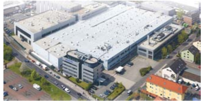
The Boll & Kirch manufacturing facility in Kerpen near Cologne, Germany
